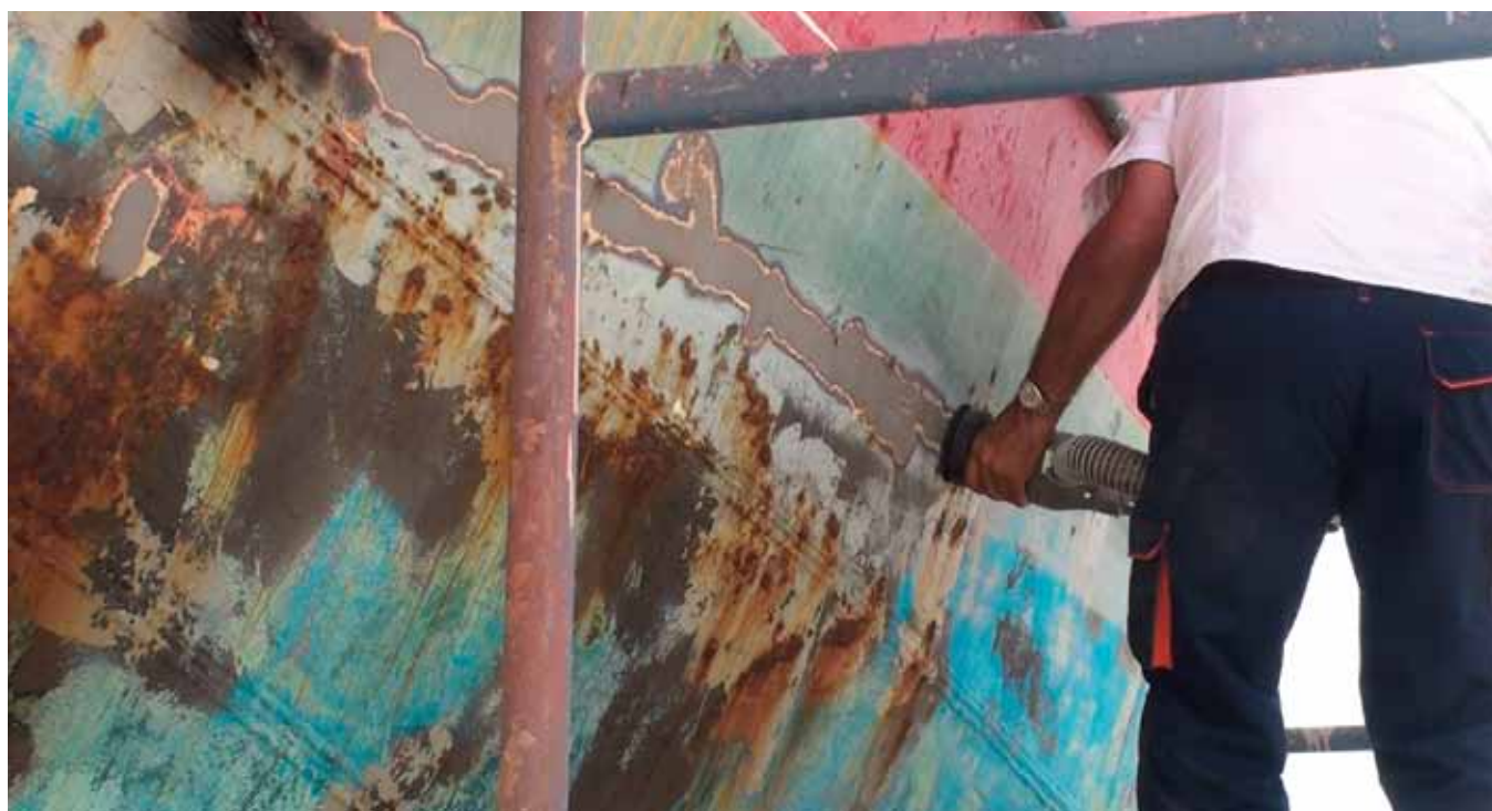
The ‘Recyship’ team trialled this safer paint removal system
